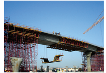
Acrow Bridge table form
