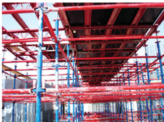
Acrow early striking system
