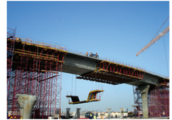
Acrow Bridge table form
