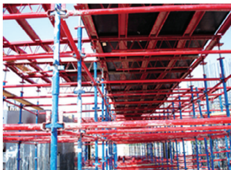
Acrow early striking system
