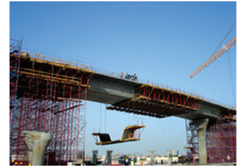
Acrow Bridge table form
